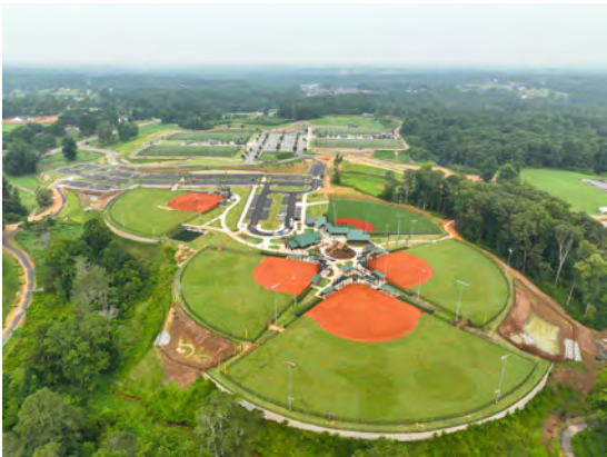
Phase 2 of the Lanierland's master plan for expansion is complete and unveiling to the public is scheduled in Mid-August 2023.
