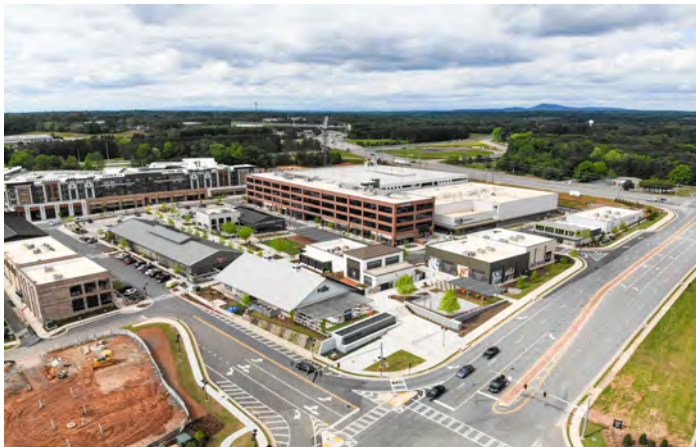
McFarland Rd/GA 400 Interchange
