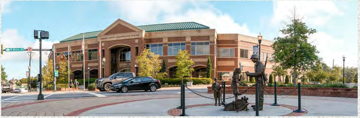
Forsyth County Administration Building
